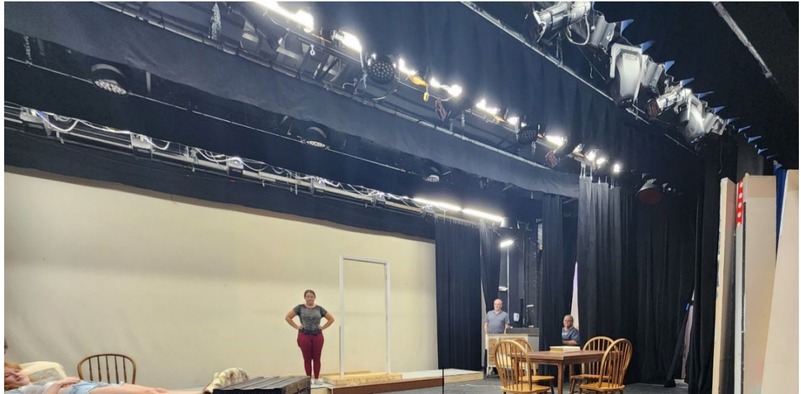
Figure 1. Shows theater light battens (2-inch steel pipes on which multiple types of theater equipment are hung (lights, speakers, flats, etc.). Also shows existing CYC hung from furthest upstage batten.
