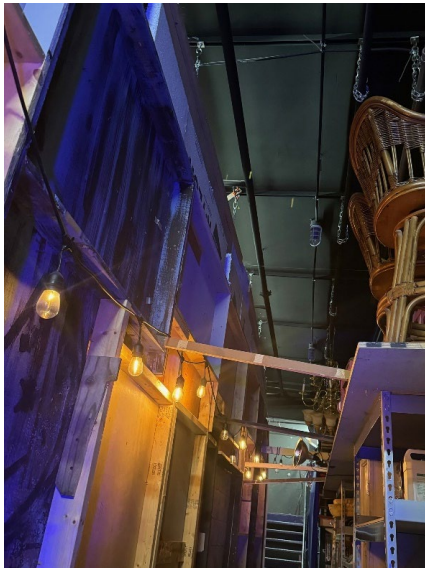
Figure 3. Shows the cyc "wall" (wood frames screwed together with luan on one side) hanging by chains from attached to a theater unistrut and one of the light battens (2-inch steel water pipes). It is further stabilized by wood struts attached to the back theater wall and being screwed to the floor. New LED "wall" will replace the cyc "wall" and hang from the same light batten.
