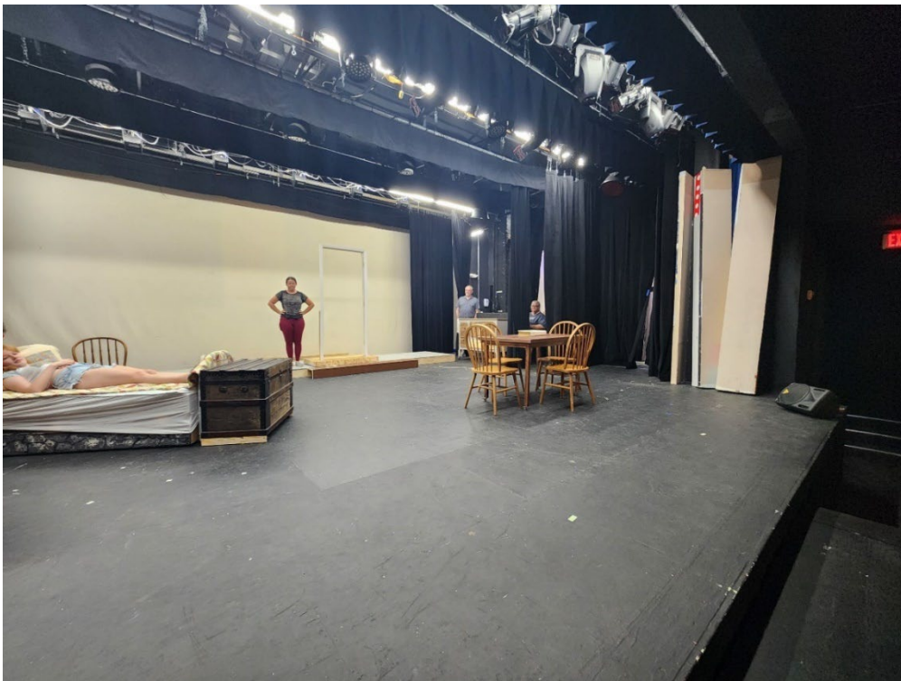
Figure 4. Shows the open theater stage with the current CYC at the rear (wood frames attached together and covered by a cream-colored fabric on the audience side, and then hung from a lighting batten) which will be replaced with the new LED CYC.
